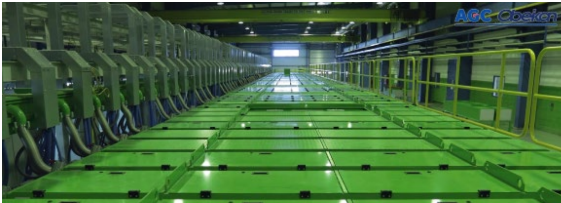
Coating equipment in AGC Obeikan
